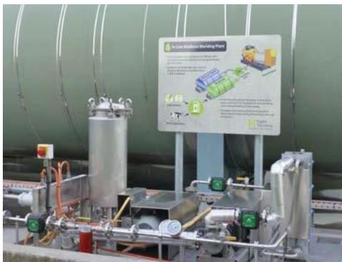
Testing the use of bio diesel as a mix with mineral diesel has lead Hydro to the view that a mix of 20% biodiesel into the mineral diesel is the best mix. Bio diesel was imported to King Island for the trial.
