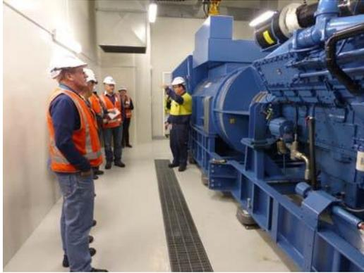
*The D-UPS provides an immediate short-term backup for the primary diesel generators – it makes sure that there is not a gap in generation when the customer demand rapidly exceeds renewable generation.*
